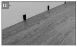
10. Once the room has been completed the spacers can be removed and the expansion gap can be covered with a skirting or a trim.
