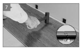
7. The use of a rubber mallet in conjunction with a tapping block can be used to fully secure the locking system. This requires no more than a tapping force.
