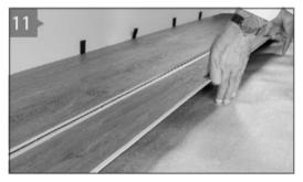
11. To disassemble the planks row by row, lift the entire row to the same angle as when being installed, the row can now be slid apart.
