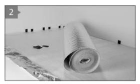
2. The use of a suitable LVT underlay not exceeding 1.5mm is recommended assisting with the installation and slight unevenness in the subfloor. To maintain an even expansion gap place spacers to give a equal distance between the wall and the plank.
