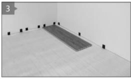
3. it is of the upmost importance that the first row is installed straightly to achieve this both rows one and two will be installed together alternating between planks at each stage, this will only need to be done for the first two rows. Row one is started with a cut down half plank.
