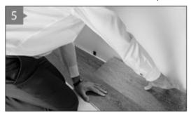
5. The second plank of row one will also be a full size long plank, once again angle the long side of this plank into the long side of row two's first plank, slide the third plank to the left so the short end meets the short end of the first plank of row one, it is then lowered to lock into position
