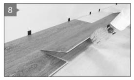
8. Continue to construct rows one and two by alternating boards to avoid any misalignment. At the end of the row measure back and cut the board to suit making sure to allow for the expansion gap. Row 3 onwards will not require this alternating method and a single row can be installed at a time.
