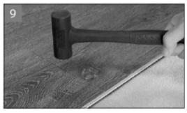
9. Continue to use the rubber mallet and tapping block to fully secure the locking system. Remember this requires no more than a tapping force.
