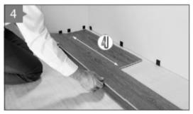
4. The first plank of row two will be a full size plank, angle the long side of row twos first plank onto the long side of plank one of row one, lower plank one of row two to lock them both together making sure there are no gaps.
